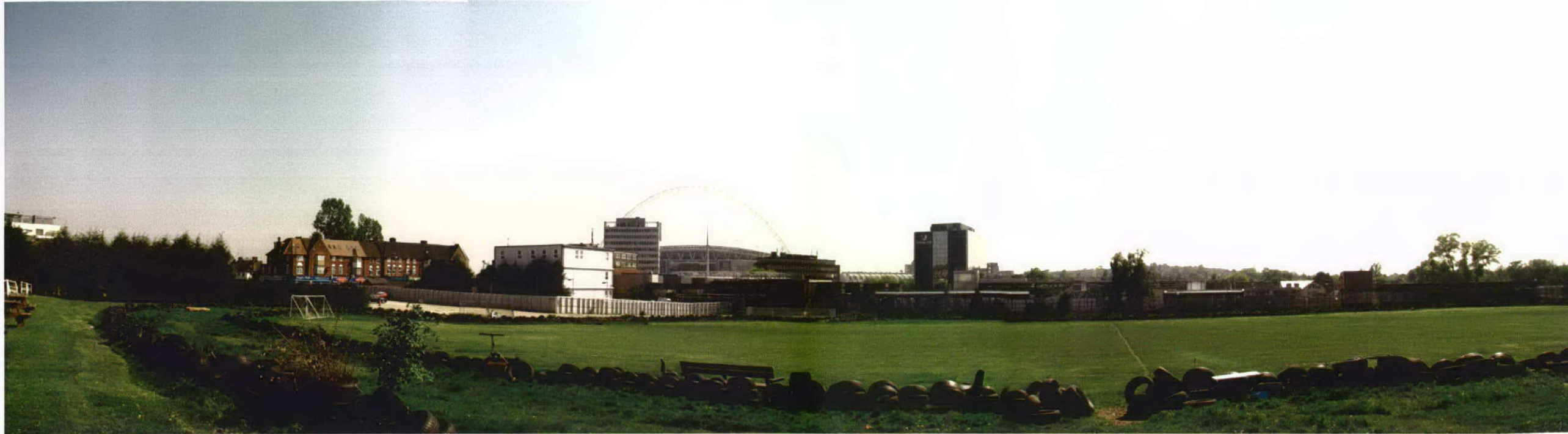
View across site to Wembley Arch
